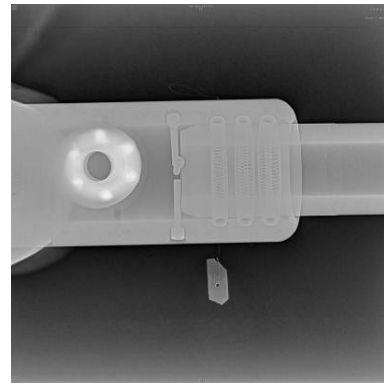
Fig. 12 The X-ray photo of a metal aluminum block on the high-voltage conductive pole inside the bus segment
