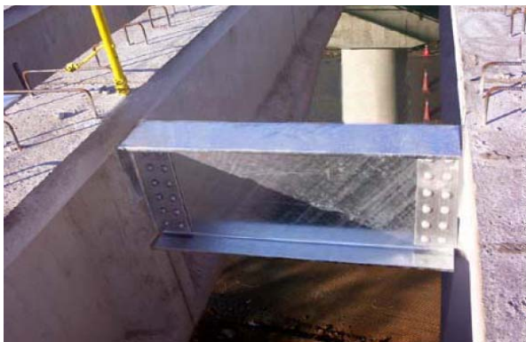
Fig. 3 Steel Cross Beam
