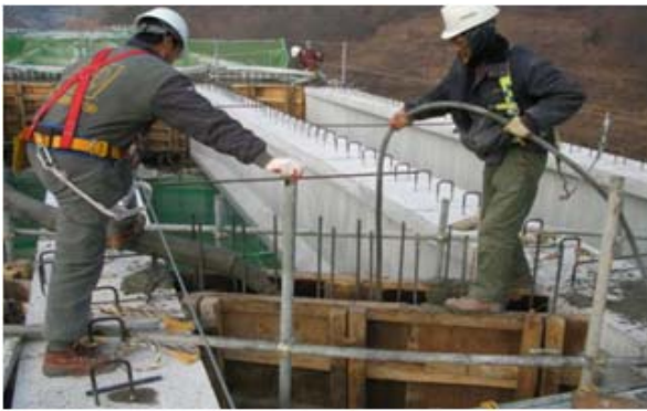
Fig. 2 Placing Diaphragm in Field
