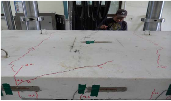
Fig. 11 Crack in ST Type
