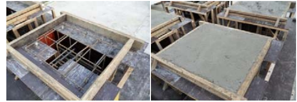
(a) Installing Bar and Cast
