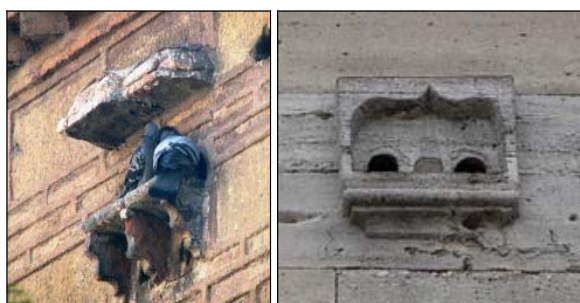
Fig. 2 Extension type dovecotes [6]
