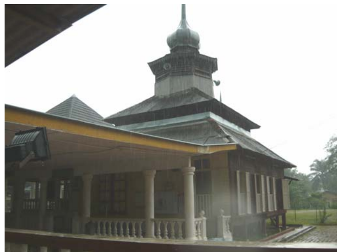
Fig. 2: Renovations and additional structure were supported to the Old Mosque of Kg. Mendun, in Negeri Sembilan.
