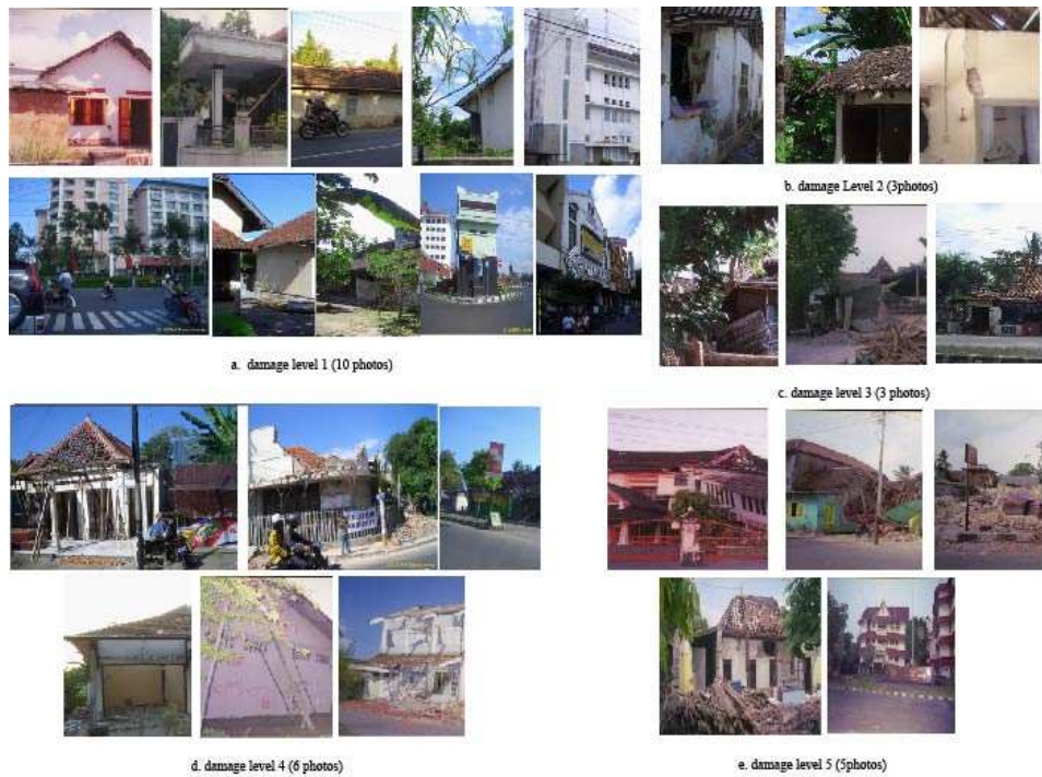
Fig. 1 Damaged photographs of masonry structure
