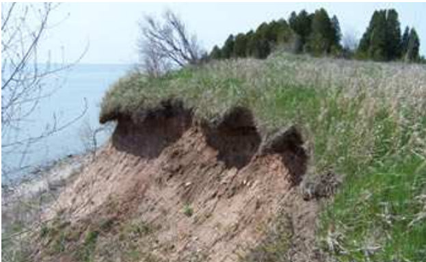
Fig. 2 Collapse of layer undercut by piping / sapping [6]
