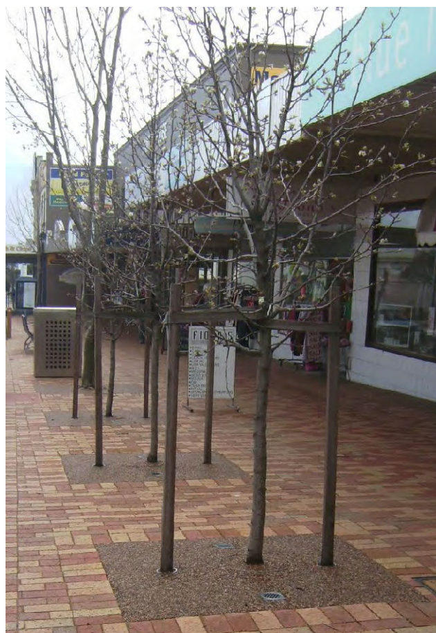
Fig. 3 In-situ WSUD Street Tree Pit
