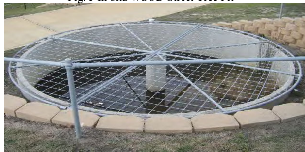
Fig. 4 Hi-Capacity Sedimentation Tank
