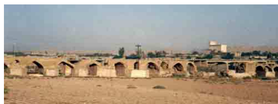
Fig. 1 Shadorvan Bridge Barrier (Dam Blocker): Different views from dam blocker
