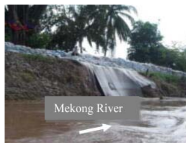
Fig. 3 Sheet-Flood erosion control work situation*
