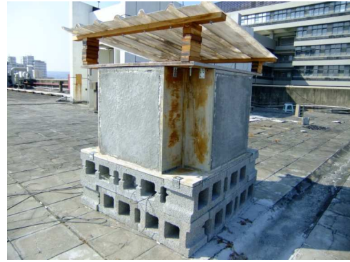
Fig. 4 Control group consisting of reinforced concrete exterior walls
