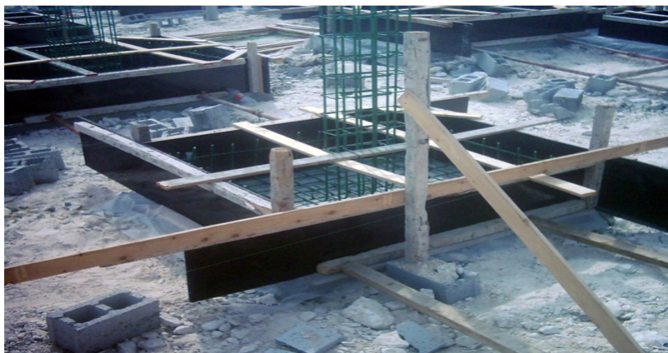
Fig. 4 Footing formwork material – Four sides
