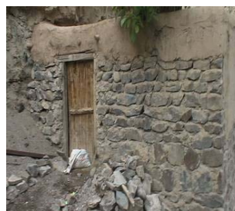
Fig. 6 Stone in the building's walls
