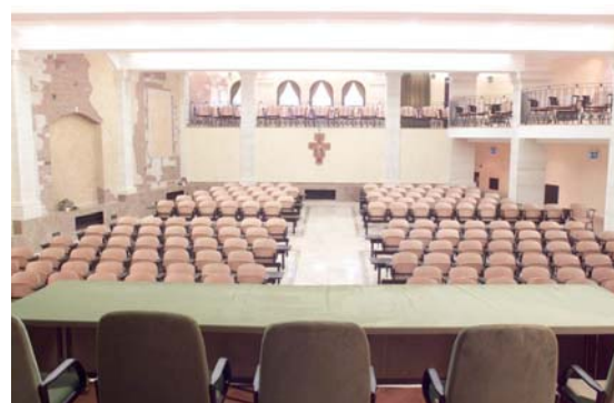
Fig. 5 View of the auditorium from the stage
