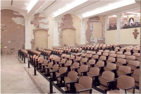
Fig. 6 View of the pit and the ceiling
