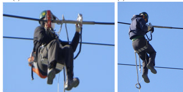
(c) Domestic line sleeve inspect method Fig. 1 Line sleeve inspect
