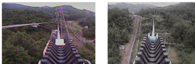
(a) Dual line test (b) Single line test Fig. 14 Actual line test on Sin-Okcheon Substation
