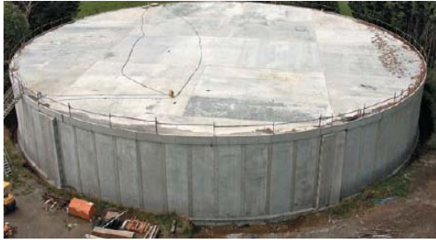
Fig. 2 Completed 20000 m 3 , pre-cast concrete reservoir.
