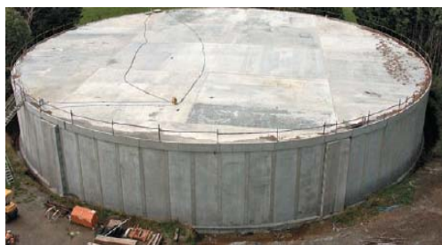
Fig. 2 Completed 20000 m 3 , pre-cast concrete reservoir.
