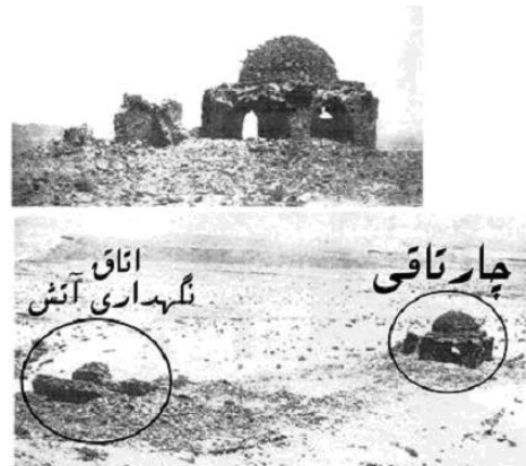
Fig.14 Cross-vault of the village “Dah Sheikh” (“Dasht-e-Ab/Baft district/Sirjan, a city in Kerman)
