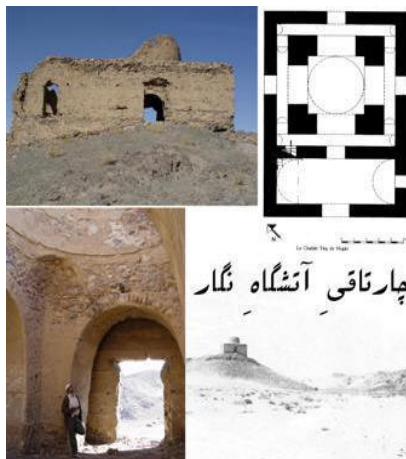
Fig.30 Plan and pictures of "Negar" cross-vault (borders of "Negar" village/southwest of Kerman)
