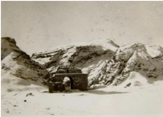
Fig.34 A plan and image taken of cross-vault "Baze-hur" in 1938 (near "Robat-Sefid"/between "Torbat Heydarriyeh and "Mashahd"). The remains of the circumferential wall which was closely around the dome-house, are destroyed and evident.
