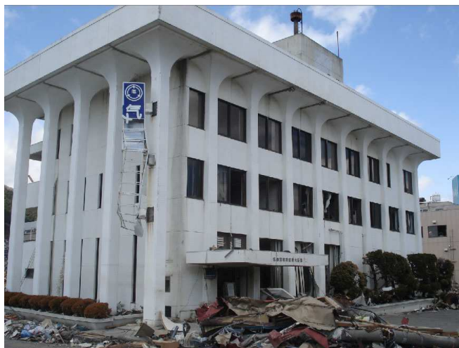
Fig. 15 RC building (Ofunato city)
