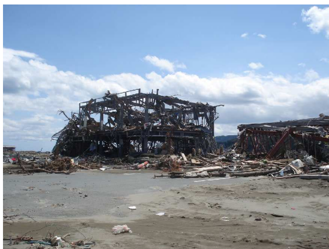
Fig. 14 Collapse of steel structure
