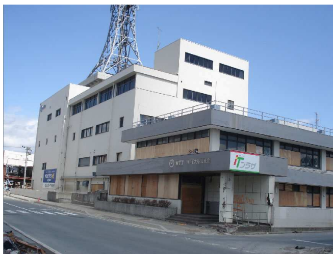
Fig. 16 Two story RC building
