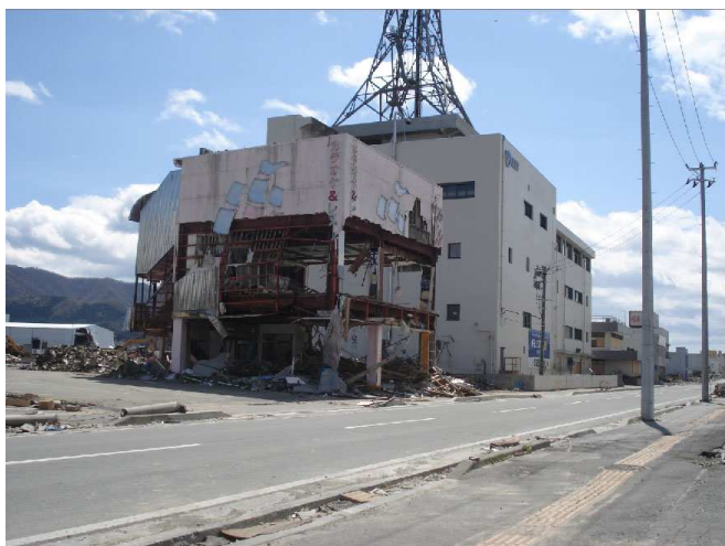
Fig. 13 Destruction of wall panels
