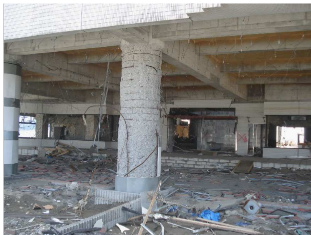
Fig. 20 Detail of RC columns
