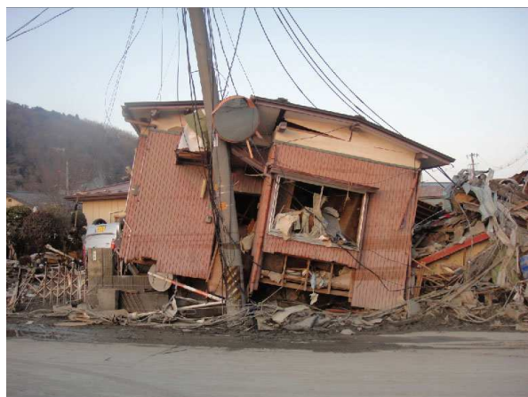
Fig. 9 Transportation of the upper floors
