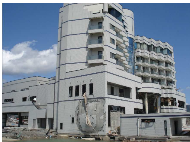
Fig. 19 RC building hotel
