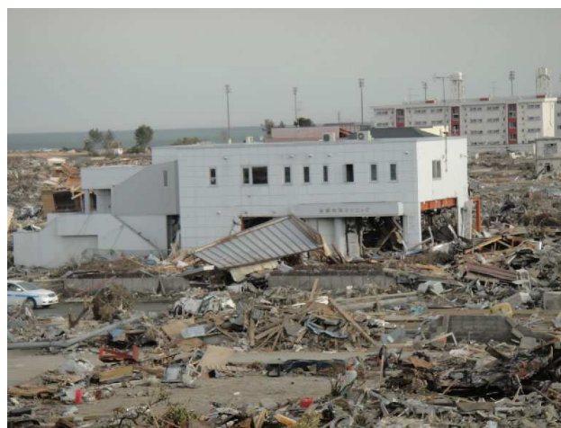
Fig. 11 Steel structure almost intact
