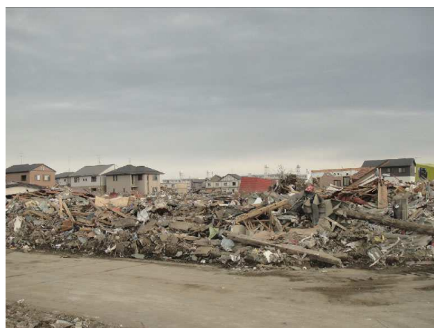
Fig. 7 General damages of wooden houses
