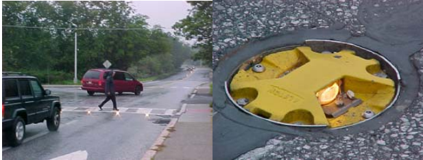
Fig. 9 In-pavement flashing warning lights in Denville [9]
