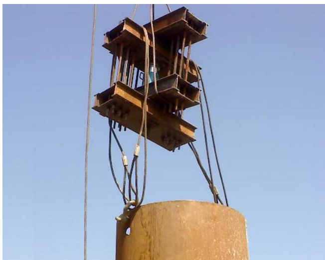
Fig. 3 Imposing tension force to pile
