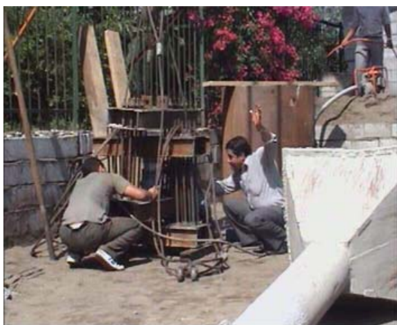
Fig. 2 Hydraulic Jack installation in the frame.
