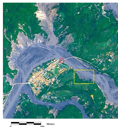
Fig.2 Destroyed bridge segment and flooded area
