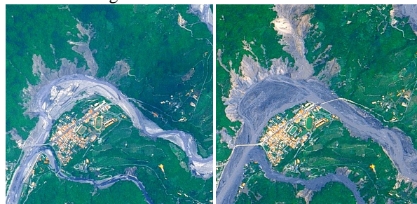
Fig.1 Baolai-2 Bridge and its surroundings before and after Typhoon Morakot strike
