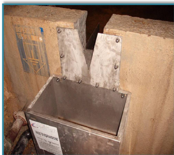
Fig. 3 Weirs used to monitor tunnel inflows
