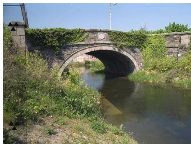
Fig. 1 Griffith Bridge – Dublin
