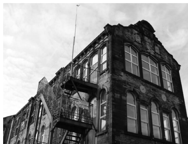
Fig. 1 Photograph of A-Block, St. Lukes Hospital, Bradford, UK
