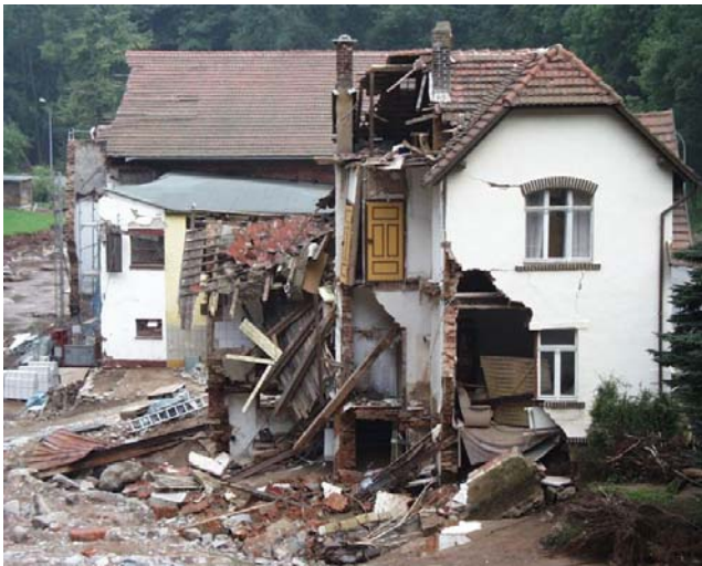
Fig. 2. Example of a close to collapse building with intact floor parts. Photo: Michael Markus.
