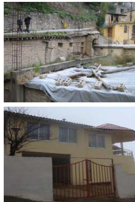
Fig. 14 New construction in staircase structure of Masouleh
