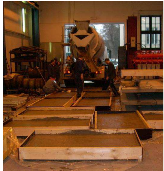
Fig. 5 Casting of specimens without inner supports
