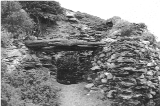
Fig. 3 Lime Kiln 1 as seen from the access path
