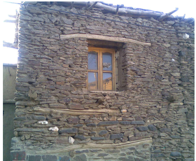
Fig. 3 using the stony thick wall in order to make the thermal insulator (Varkaneh village, Hamedan, Iran)
