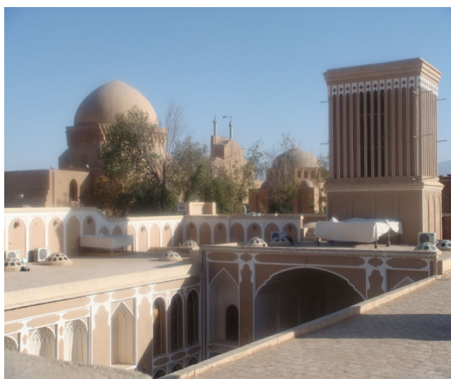
Fig. 1 The way of yard position in the centre and using the air hole (Yazd, Iran)
