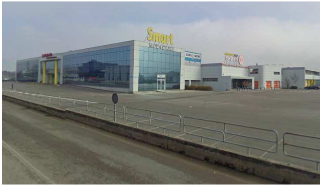
Fig. 3 South-West view of the building
