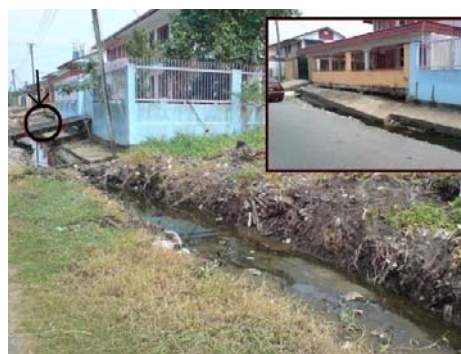
Fig. 1 Housing area on low-lying peat soil ground, Jalan Lai Chee, Sibu.
