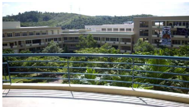
Fig. 14: A depiction of the ground and surrounding area corresponding to model III. Notice the foliage, which may well have shadowing effects on radio paths between a transmit spot on the ground area and the receiver located up at level four of building.
