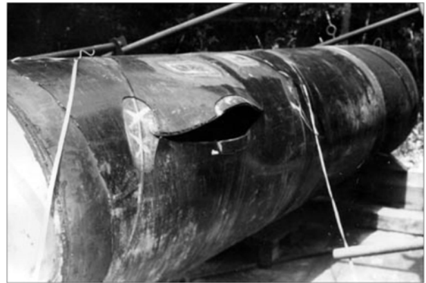
Fig. 6 Burst initiated on the slit B with a fatigue crack
