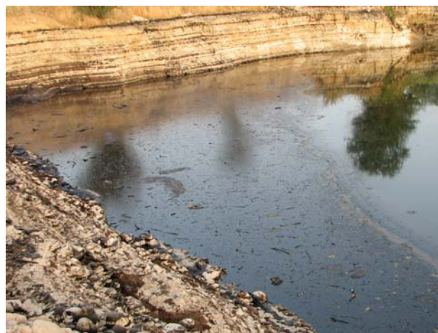
Fig. 2 Storage of effluent of sugar factory in the basins net to the Beshar stream
