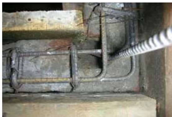
Fig. 6 Reinforcement Details @ corners
