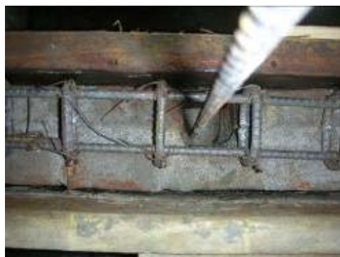
Fig. 5 Reinforcement Details @ junction
