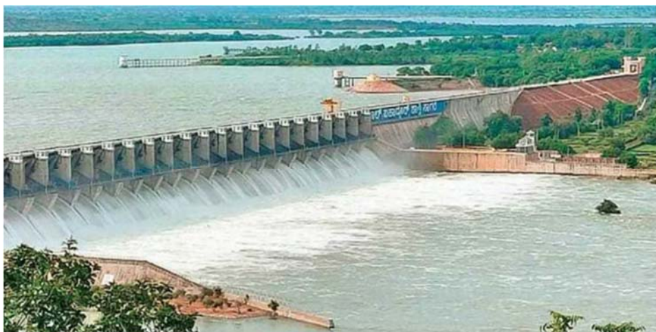
Fig. 2 Overview of the Almatti Dam
