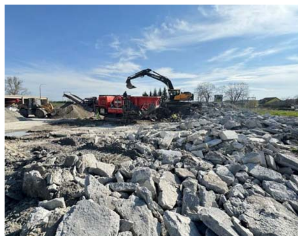
Fig. 2 Demolition concrete processing and aggregate crushing
