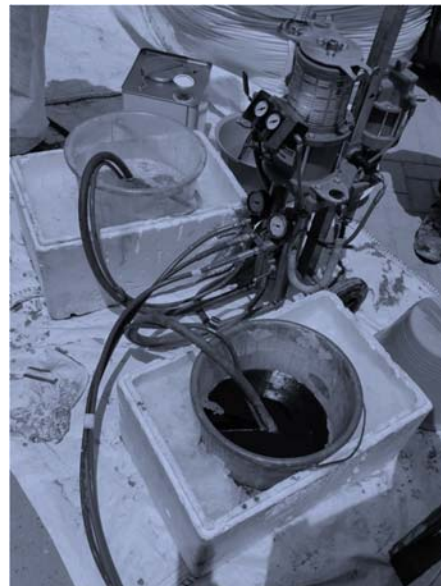
Fig. 2 Expanding resin injection application during hot temperature with storing the components in ice boxes
