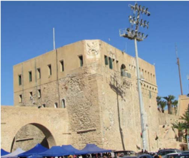
Fig. 10 An external view of St. Gorge Tower [1]
