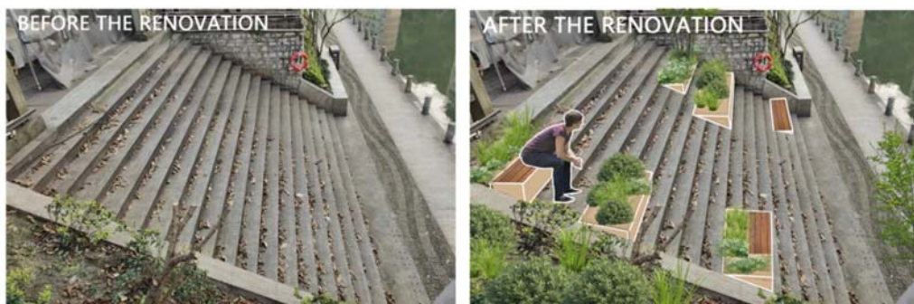
Fig.14 Waterfront staircase renovation
