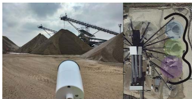
Fig. 4 Calculation of the volume of stockpiles automatically through the use of cameras
