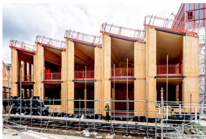
Fig. 8 The installation process on the site [34]
