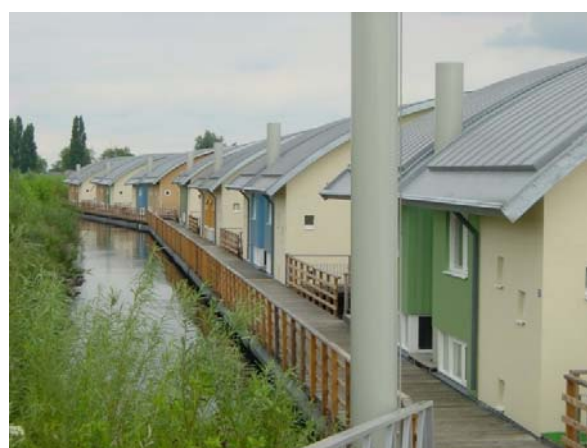
Fig. 5 View of the Floating houses Maasbommel [12]
