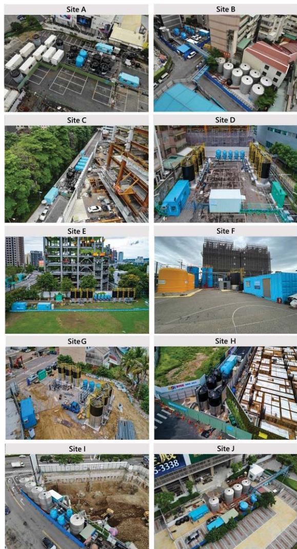
Fig. 3 Temporary Groundwater Treatment Project configuration
