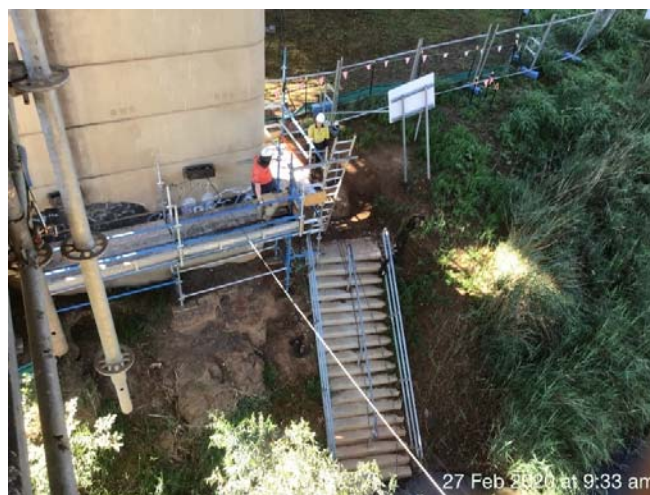
Fig. 12 Installation of diagonal restraints
