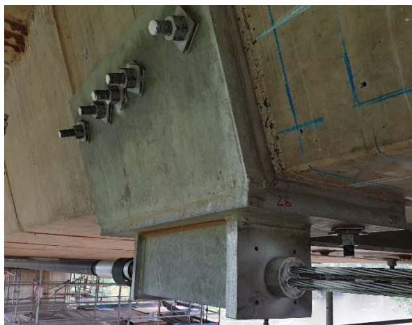
Fig. 13 Installation of anchor pods and shear keys
