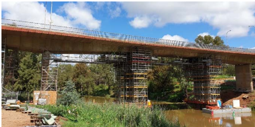
Fig. 11 Construction of the new piers
