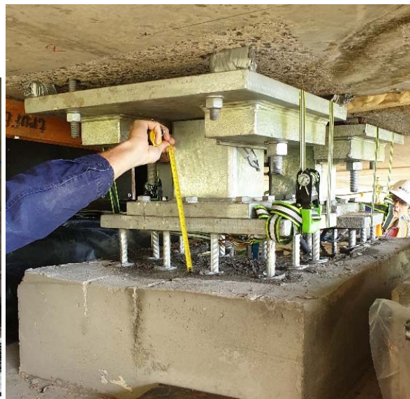
Fig. 13 Installation of anchor pods and shear keys
