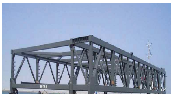
Fig. 3 Case study 1- Trestle module
