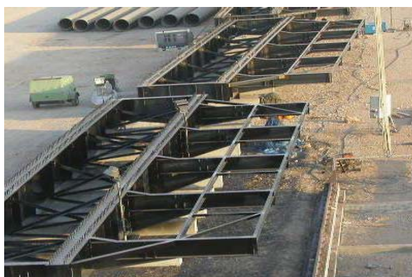
Fig. 4 Case study 2: Superstructure girder assembly in project yard
