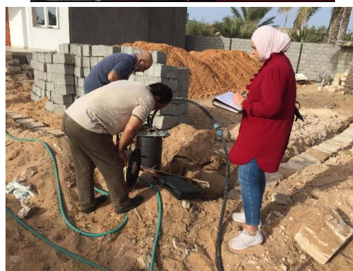
Fig. 3 Field work (Collection of samples and water level measurements)
