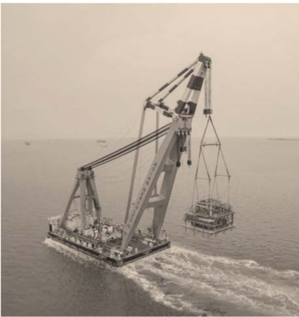
Fig. 15 Sheer leg cranes [29]
