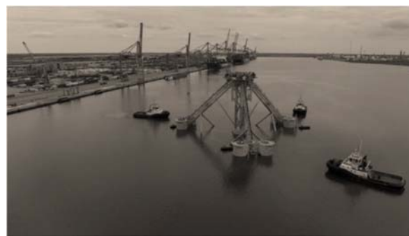
Fig. 4 TLP sub-structures in harbour [17]
