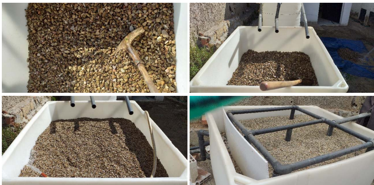
Fig. 4 Refilling of the vertical flow filter
