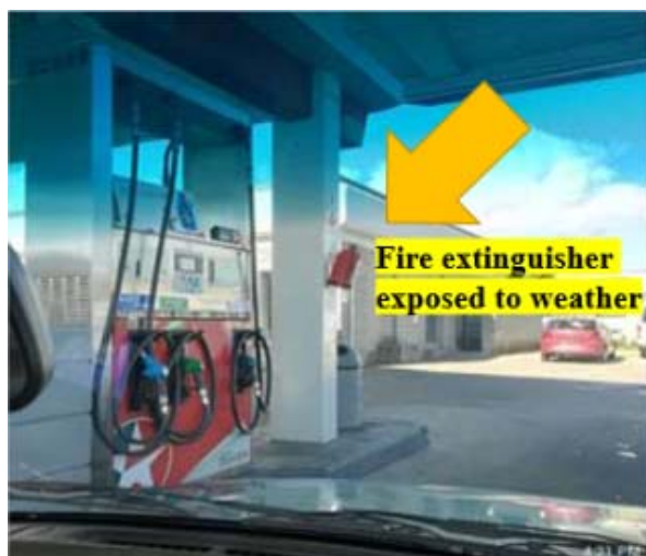
Fig. 11 Unprotected Fire Extinguisher at petrol station #6 in Stellenbosch
